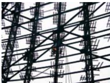
Extensive Welding. Array of field-welded connections possible with low-cost work force. (Photo courtesy of SETEC TPI)
