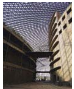
Indoor Space. Arching steel trusses welded in place resemble ladders that converge on a compression ring. They create a soaring indoor atrium shared by
