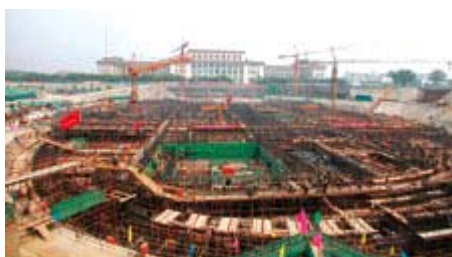
Deep Excavation. Dewatering removed 28, 000 cu m of water per day. (Photo courtesy of SETEC TPI)
