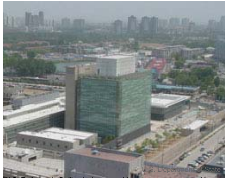
U.S. Embassy in Beijing is the second-largest ever constructed by the U.S. Dept. of State.
